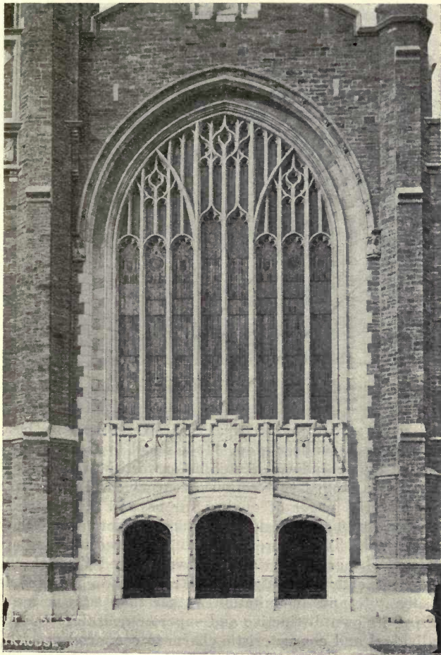
FIG. 3—ENTRANCE AND WINDOW TRIM OF CONCRETE STONE, BROADWAY PRESBYTERIAN CHURCH, NEW YORK CITY—ONONDAGA LLTHOLITE CO.
